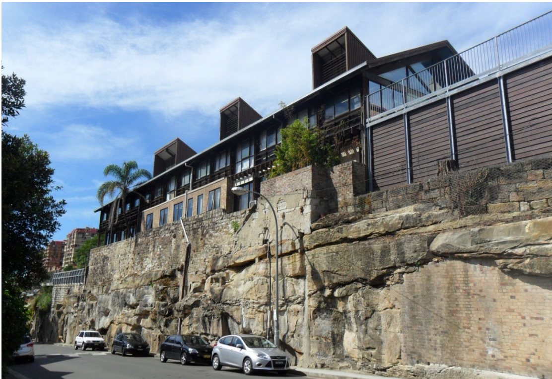
Figure 1: Calidad Building at 163 Brougham Street, Woolloomooloo, as viewed from McElhone Street
